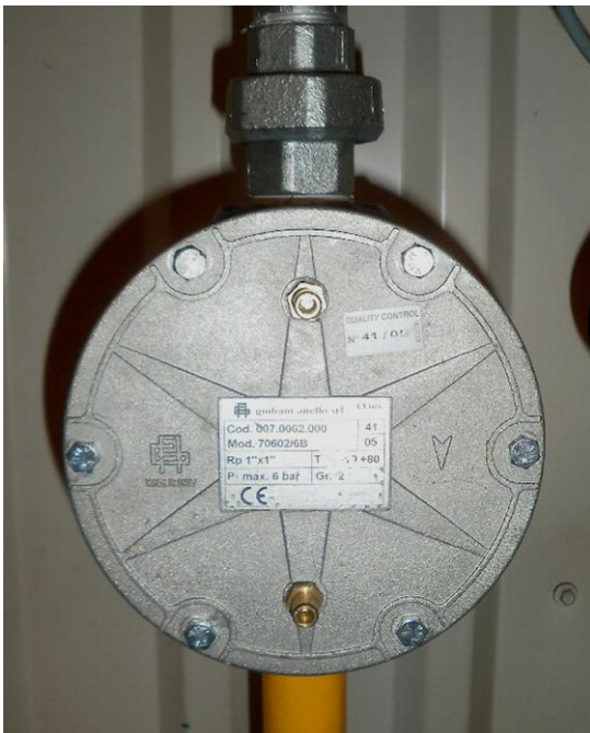
Sele 1.5 Gaasifilter
