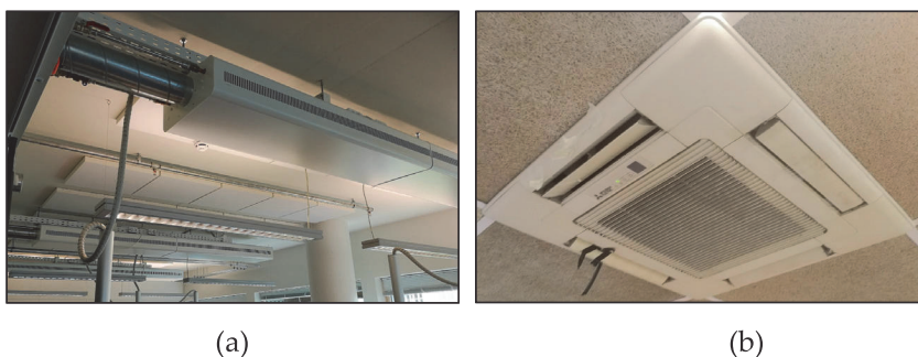
Figure 3. Possible air flow obstacles with open active beam solution (a); modified airflow distribution with fan coil unit (b).
