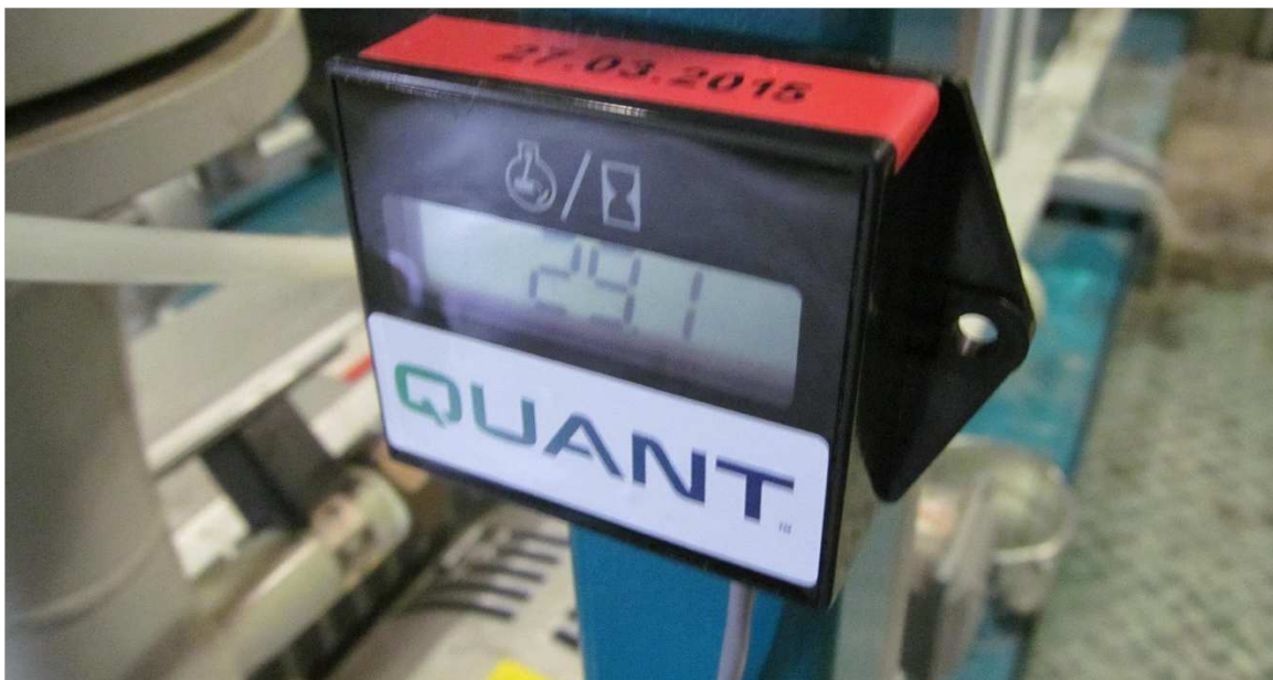
Figure 6.4 Hour counter for electric motor
