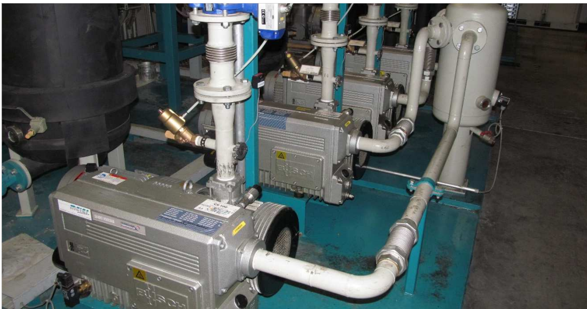
Figure 8.1 Rotary vane pumps
