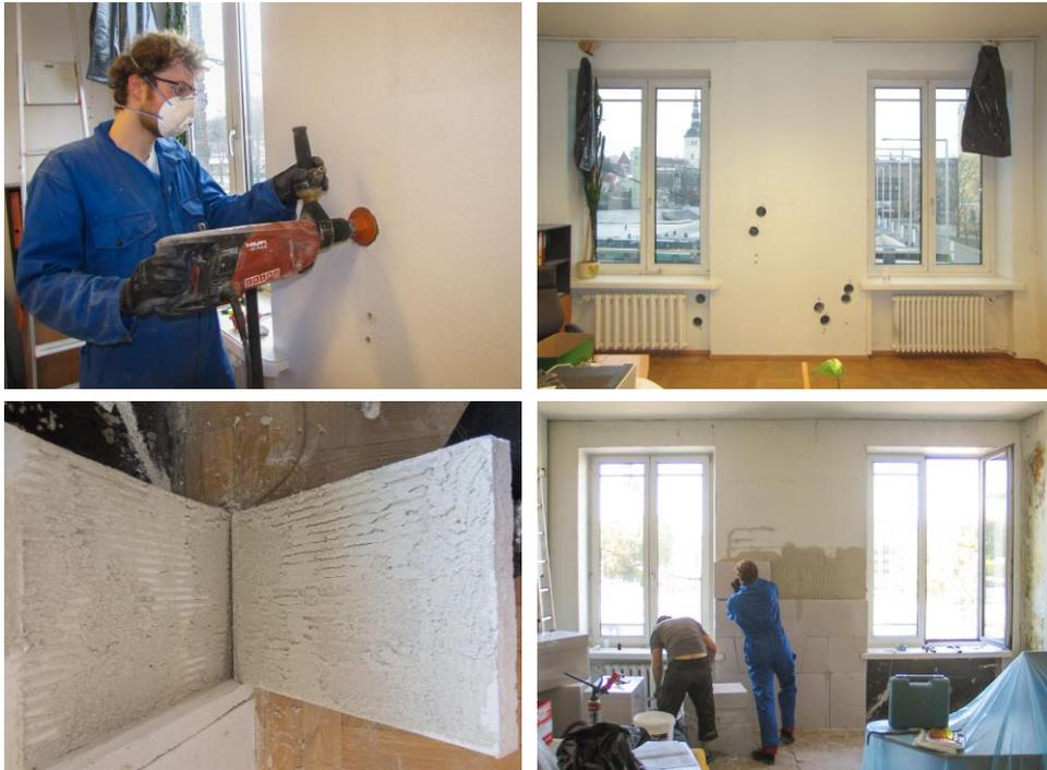
Figure 16 Sampling of the original wall to specify its structure (top left). Original wall after sampling (top right). It is relatively easy to leave air channels behind the insulation due to bad workmanship, wrong tools, too stiff mortar etc. (bottom left). Installation of insulation boards (bottom right).
