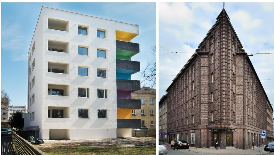
*Figure 1 Exterior insulation is the most appropriate solution to reduce heat losses through walls for most of the buildings built during the second half of the 20<sup>th</sup> century (left). However, it cannot be used if the façades are valuable (right) and one of the alternatives is the hygrothermally risky interior insulation. Source of photo on the right: Wikimedia commons user "lifar", CC BY-SA 3.0 EE.*
