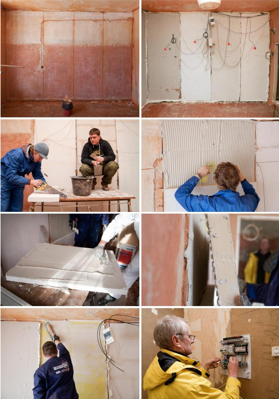
Figure 12 Top row: test wall before (left) and after (right) the installation of insulation and measurement equipment. Bottom 3 rows: different stages of the process.
