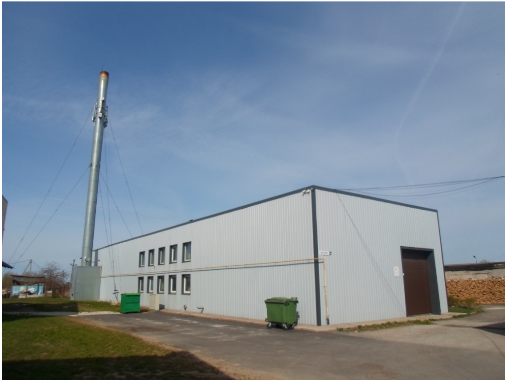
Figure 3.1 Olgina boiler house outside
