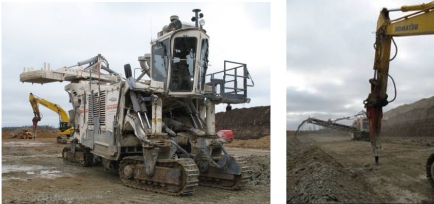
Figure 7. Wirtgen SM 2500 at Põhja-Kiviõli Open Cast mine (2006) with hydraulic rock breaker
