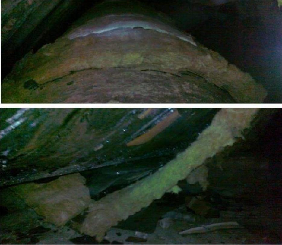
*Figure 25 Old pipes with mineral wool and tar paper insulation. The packed insulation on the top and sagging on the bottom.*
