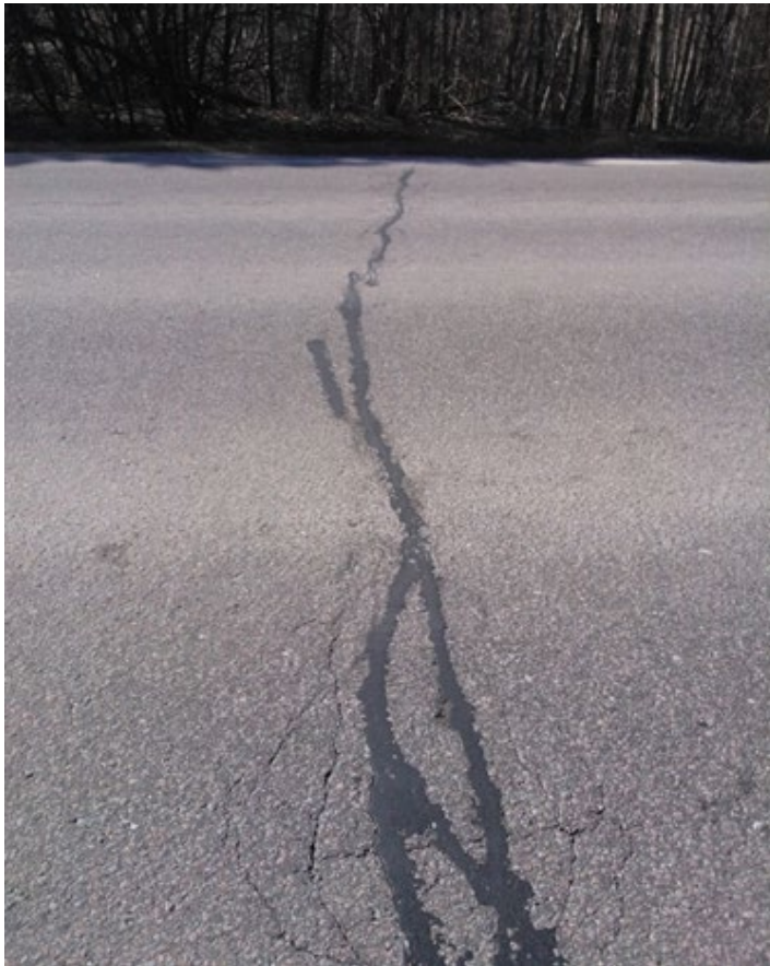
Figure 2. Pavement low temperature transverse cracking with secondary fatigue cracking adjacent to crack. Fatigue cracking is most probably caused by discontinuity in pavement structural integrity and water penetration into the subbase and subgrade.
