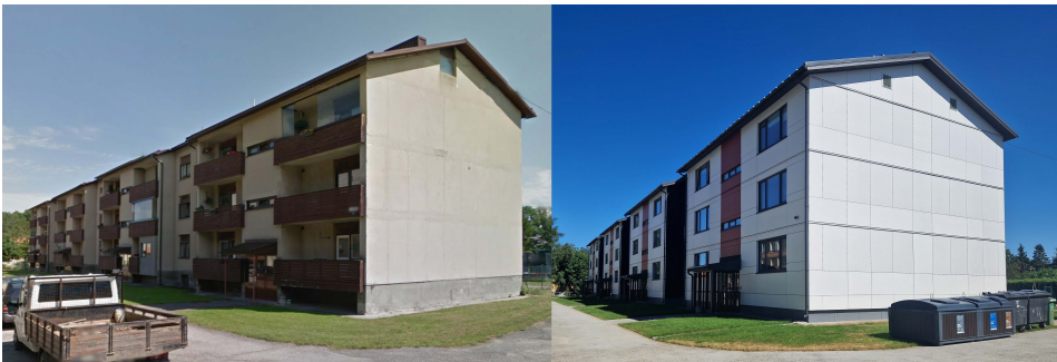
Figure 2. Typical apartment building from the housing crisis following the Second World War. Left before and right after deep renovation.
