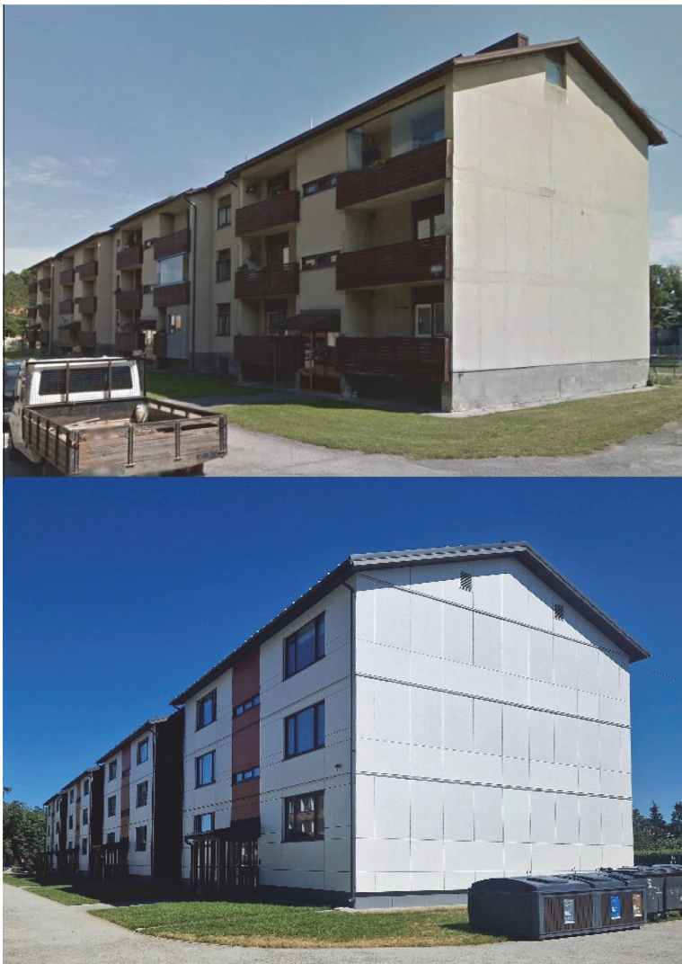
Fig. 1. Case study building – before (above, built 1986) and after (below, renovated 2021) the renovation.
