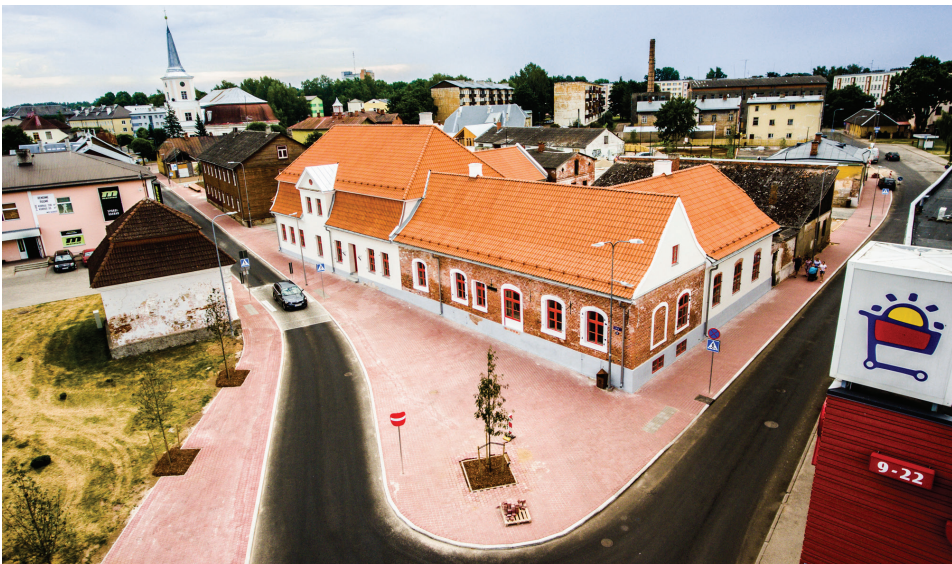
Figure 16. The cultural monument at Riia 5 after partial restoration (Valga municipality)
