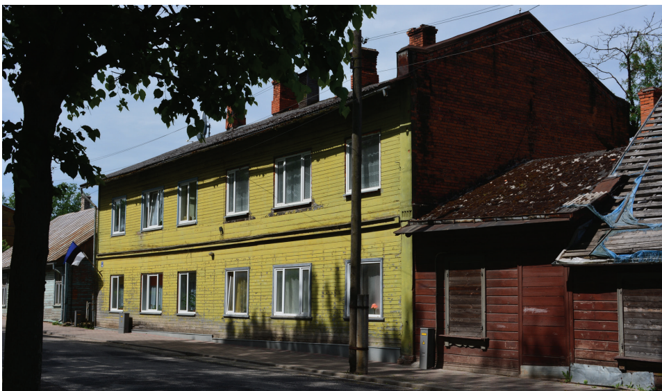
Figure 5. A typical apartment building from the first period of growth (author)
