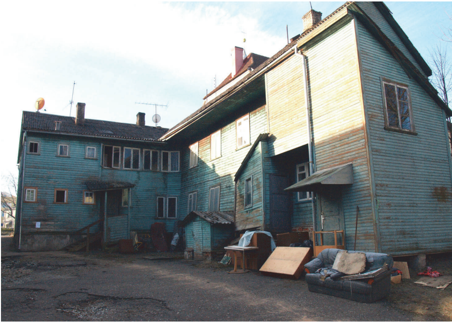
Figure 6. Kesk 20 apartment building before demolition.
