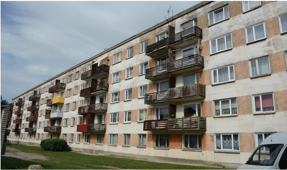
Figure 6. A typical apartment building from the second period of growth (author)
