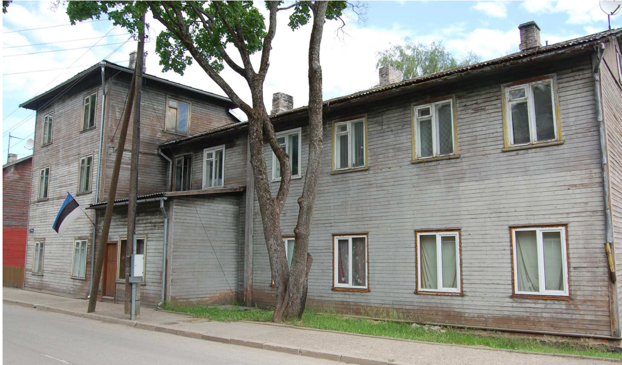
Fig.2. E. Enno 2 apartment building before demolition (authors, 2015)
