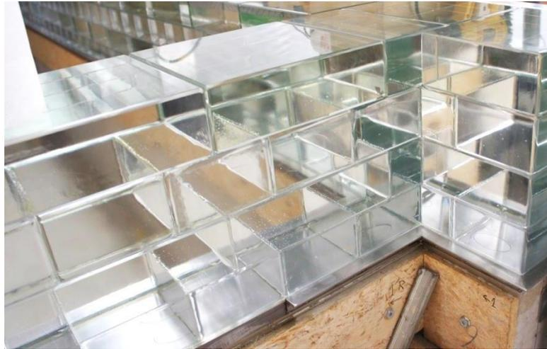
**Figure 35.** Glass block masonry system with transparent adhesive on horizontal surfaces and sealings on edge joints.
