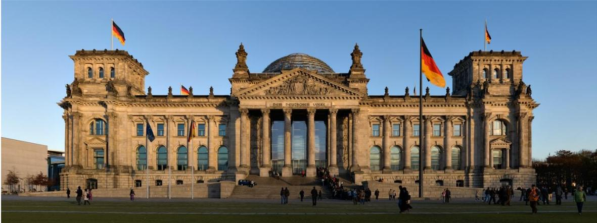
**Figure 20.** The Reichstag, German parliament building. The historic house is redesigned by using structural glass in façade and dome construction [45]
