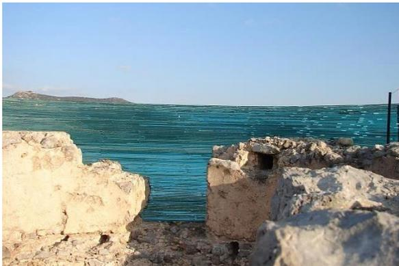
**Figure 26.** Multiple layers of float glass used to rebuild the ruined part of the mill [51]
