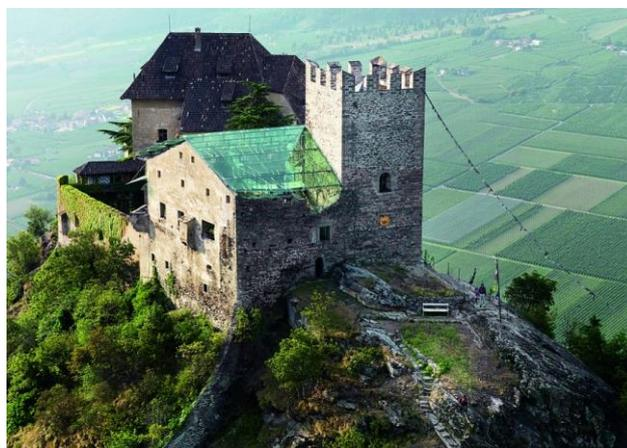
**Figure 21.** The Juval Castle in South Tyrol with its glass roof on the north wing [47]
