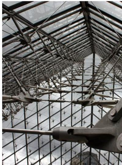
**Figure 16.** Cable truss system in Louvre Museum Glass Pyramid, France [37]
