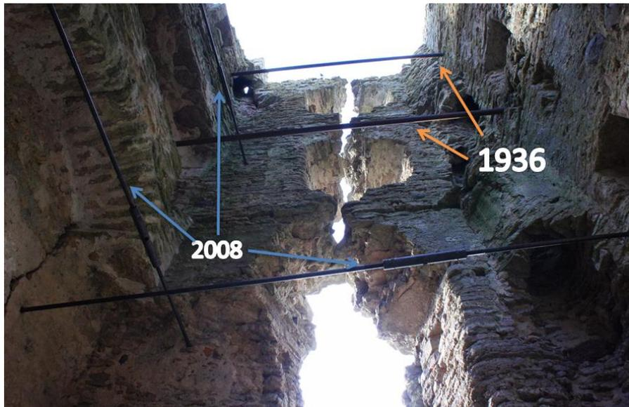
**Figure 33.** Steel anchors mounted into the SW tower to stabilize the wall movement
