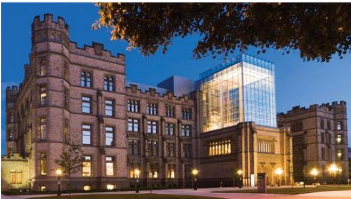
**Figure 18.** The rehabilitated Victoria Memorial Museum Building with new iconic hanging structural glass lantern[42]
