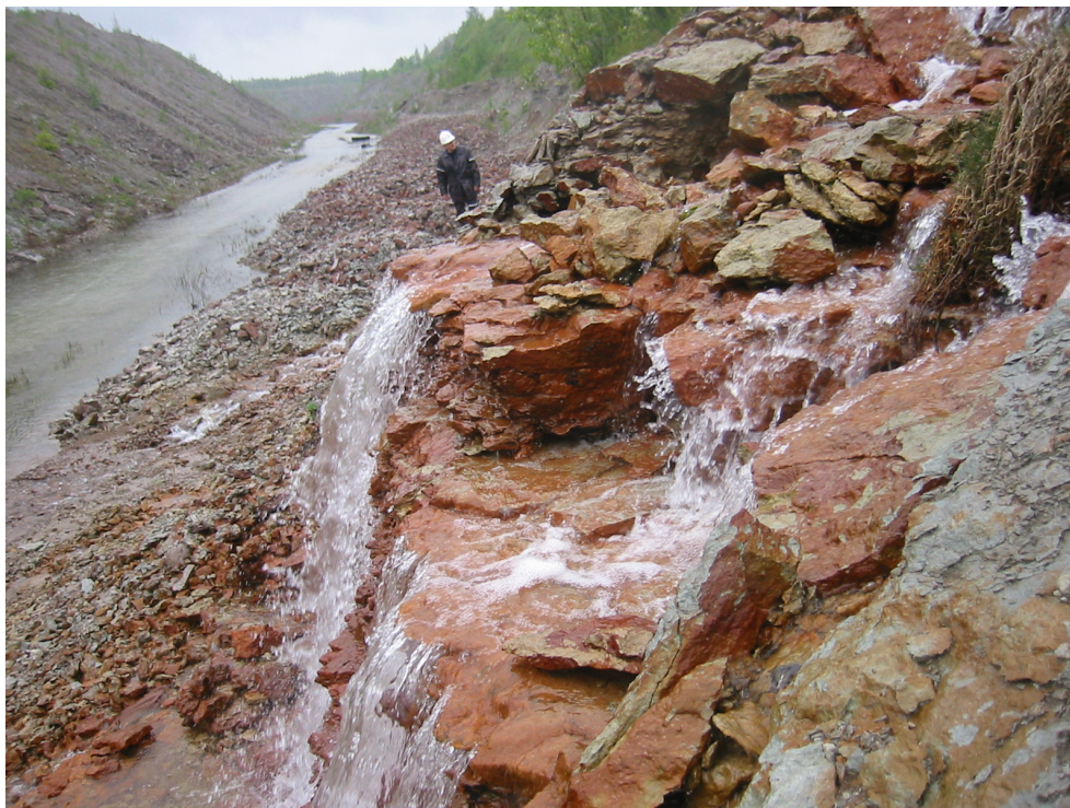
Fig. 3 Water inflow into Aidu open cast from the side of Kohtla closed underground mine
