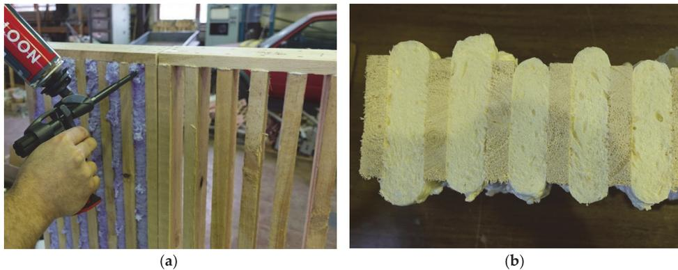
**Figure 2.** Filling the joints in a wooden frame (a) and example of a cross section (from above) of a frame with filled joints (b).
