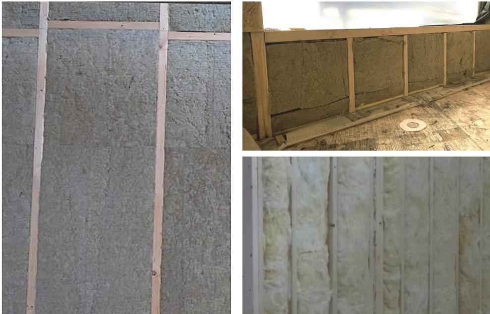
276 *Figure 6. Ideal workmanship (left) and typical non-idealities (right) for a timber framed*
