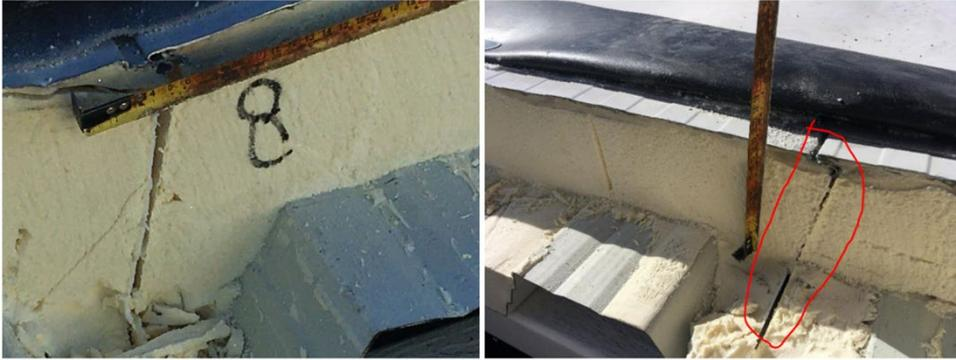
Figure 34. Penetrating air cavity formed due to aging and cyclic thermal expansion and shrinkage in the roof insulation layer.
