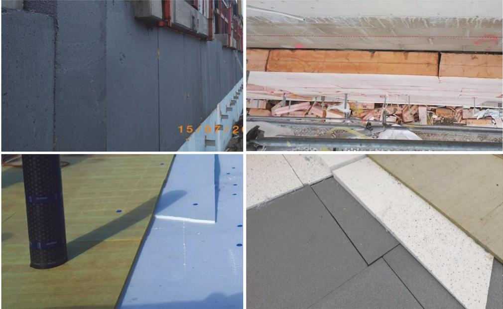
307 *Figure 8. Ideal workmanship (left) and typical non-idealities (right) for rigid insulation boards*
