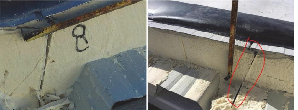
319 *Figure 9. Penetrating air cavity formed due to aging and cyclic thermal expansion and*
