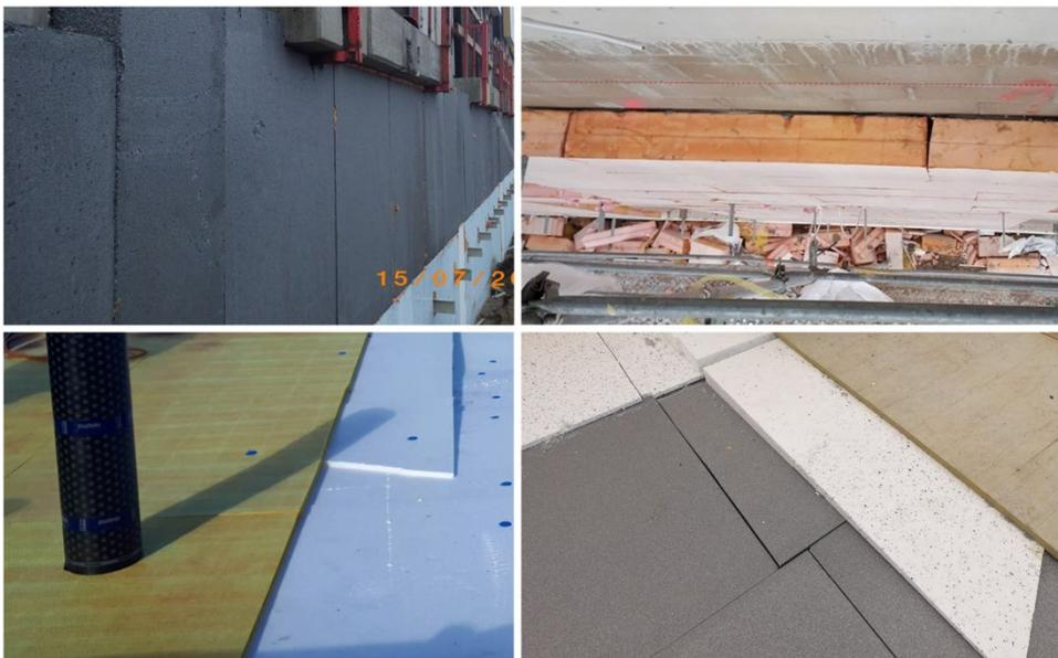
*Figure 33. Ideal workmanship (left) and typical nonideality (right) for rigid insulation boards of walls (above) and roof (below).*
