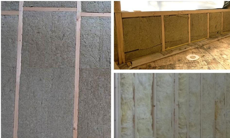
*Figure 31. Ideal workmanship (left) and typical nonideality (right) for a timber frame construction with mineral wool insulation batts.*
