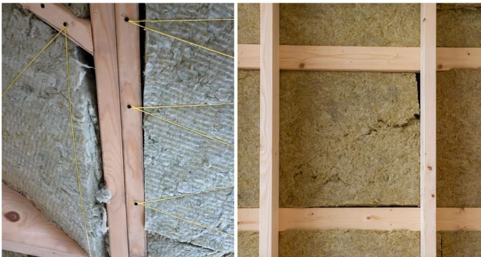
*Figure 32. Non-acceptable installation of mineral wool insulation batts in timber framed construction.*
