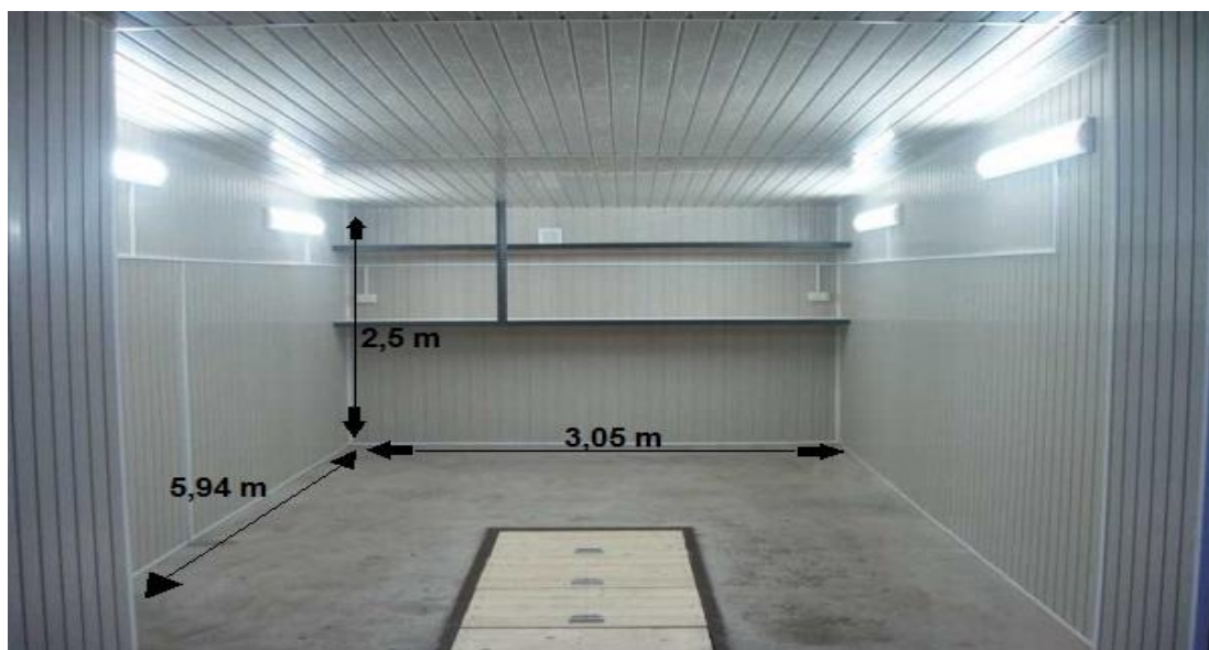
Fig.6. Dimensions of the painting chamber
