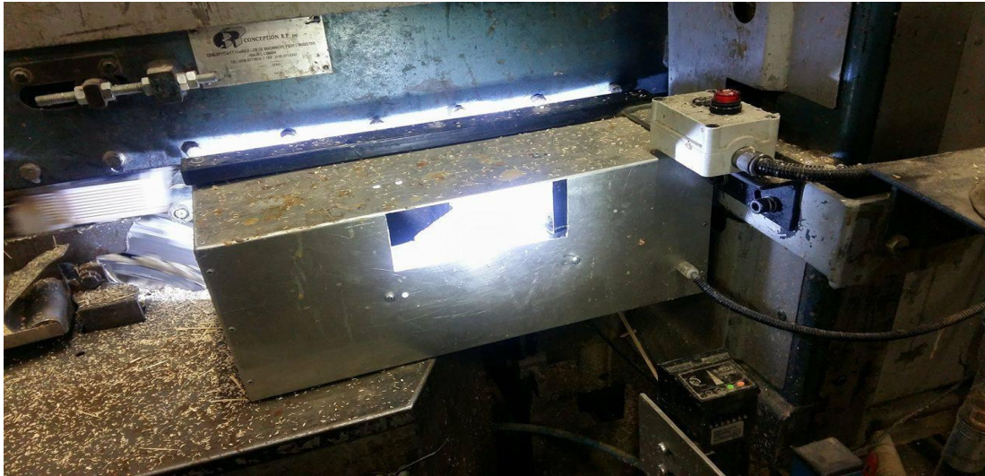
Figure 4.3 Installation of Box and accessories
