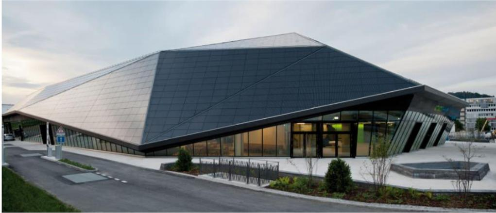
**Figure 5.** Umweltarena Spreitenbach (Switzerland 2012): an example of a 203% PlusEnergy building achieved by means of a customized 750 kWp full-roof BIPV skin consisting of c-Si panels with an antireflective glass (Architect: René Schmid Architekten; System provider : 3-S Photovoltaics, Meyer & Burger Group; Photo: Bruno Helbling)
