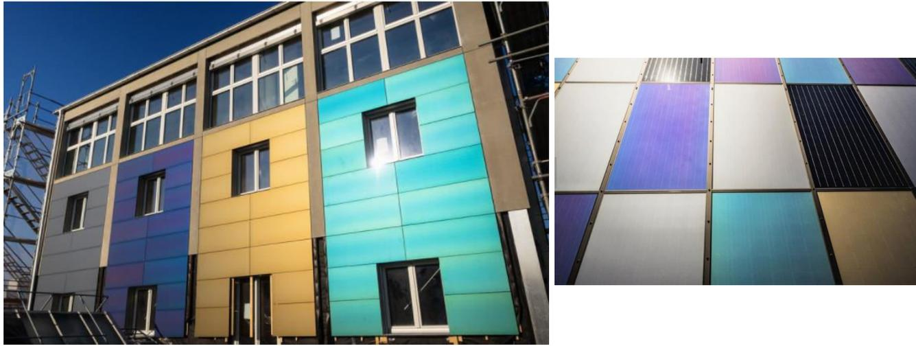
**Figure 13.** Basel, Switzerland, Kromatix™ Glass: Grey, Blue, Blue Green and Gold, Surface Area: 159 sqm, Installed capacity: 24 kWp (Source: SwissInso).
