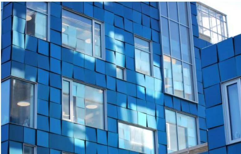
**Figure 12.** Location: Copenhagen, Denmark, Kromatix™ Glass: Blue Green, Surface Area: 6,048 sqm, Installed capacity: 1,030 kWp (Source: SwissInso).
