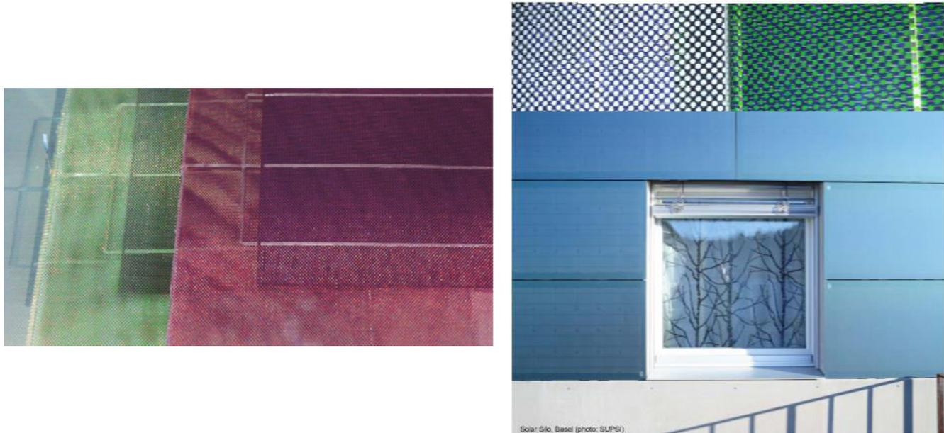
**Figure 15.** PV cells with ceramic digital printed front glass (Source: Left: SmartFlex Solarfacades), Right: Solar Silo (Basel)).
