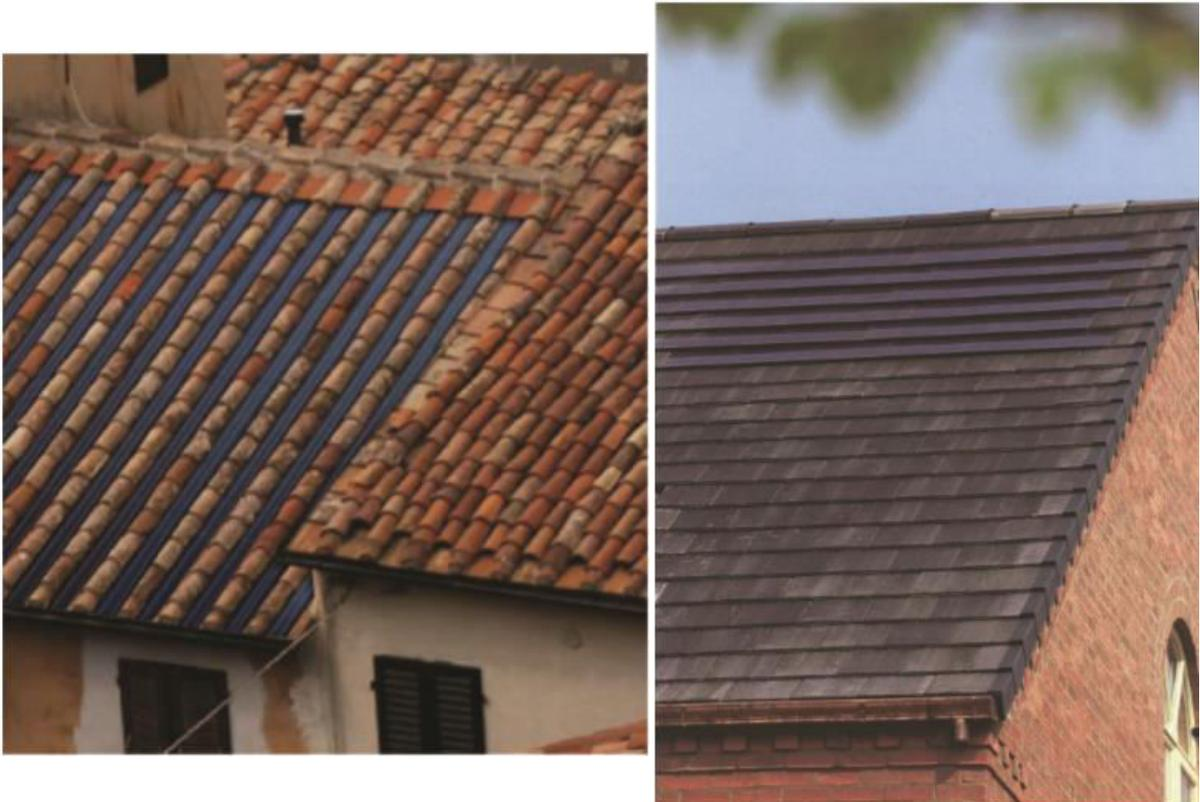
**Figure 7.** Left: Vertical tile BIPV solution. System provider: Hemera, Right: Solar shingles. System provider: Solar Century Corp. (Source: P. Heinstein et al., 2017).
