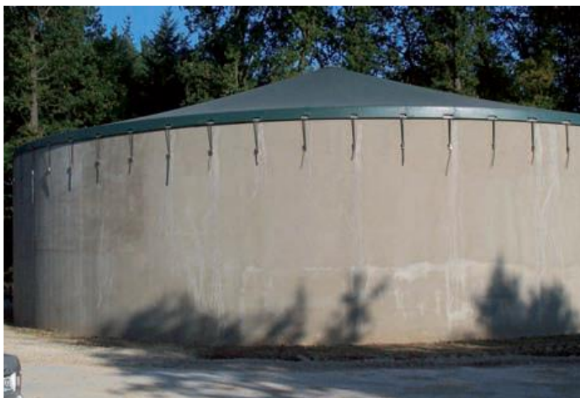
Figure 3.6 Covered digestate storage tank (reproduced from Lukehurst, Frost, & Seadi, 2010)
