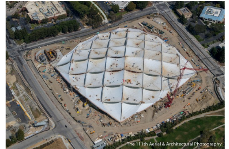
Pilt 20. Google HQ katuse ehitamise progress, Metalocus 2019 (allikas: https://www.metalocus.es/en/news/big-heatherwick-studios-google-headquarters-roof-construction-progress )
