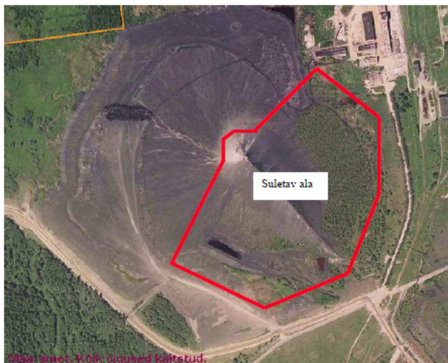
Fig. 4.1.2. Orthophoto of the Kivõli western landfill. The portion of the landfill determined for closing up (17 ha) has been surrounded by a red contour (Tööstusjäätmete ja...2007).
