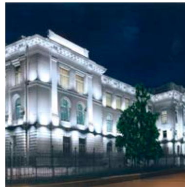
Figure 47. LUCIA pilot site at St. Petersburg (photo provided by SPbPU).
