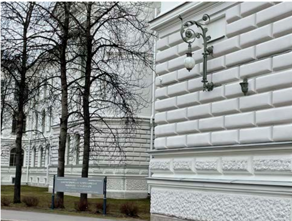
Figure 30. Historical public lighting at the SPbPU main building (photo by Yury Nurulin).
