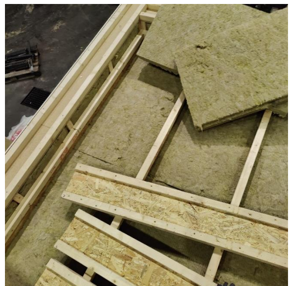
Figure 4.4 LEFT: Ceiling without insulation; RIGHT: Insulating the cavities
