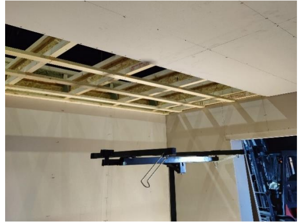
Figure 4.3 LEFT: Erected walls; RIGHT: Ceiling gypsum installation
