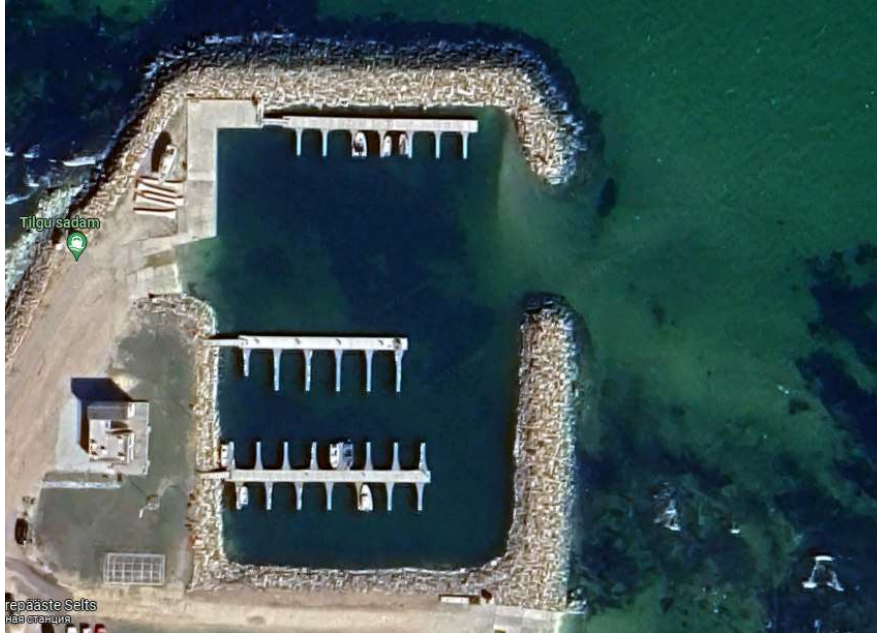
Figure 34. 'Tilgu' port picture from the satellite on the Google Maps [20].
