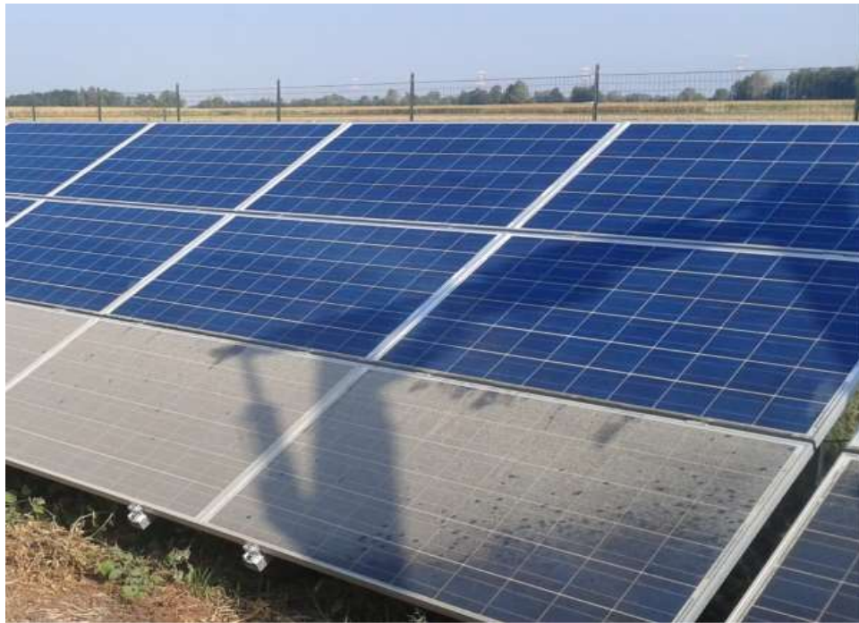
Figure 1.7. PV panel soiling [19]
