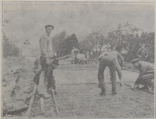
Joon. 114. Betoontee ehitamine.
