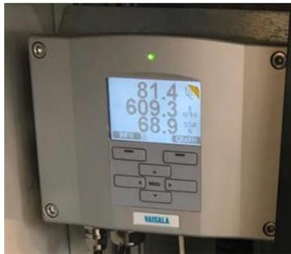
Figure 2.9 Vaisala Dew Point Transmitter DMT346
