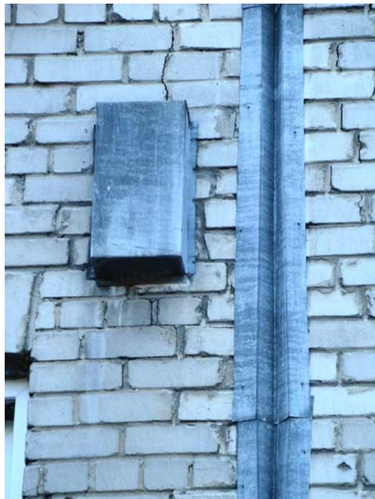
Figure 6 Breaches in building construction up to 0,5m have been covered with metal plates. Pärnu, Tallinn rd.1; photo by Tõnu Kütt
