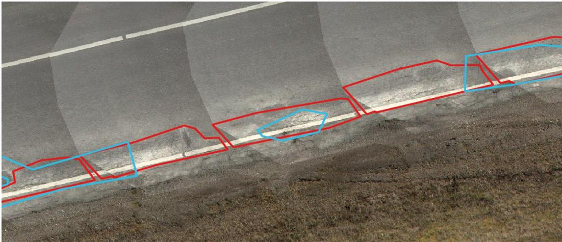
Figure 8.21 Example of predictions of network cracking compared to the annotations. The blue denotes the annotated defects and the red the predictions.
