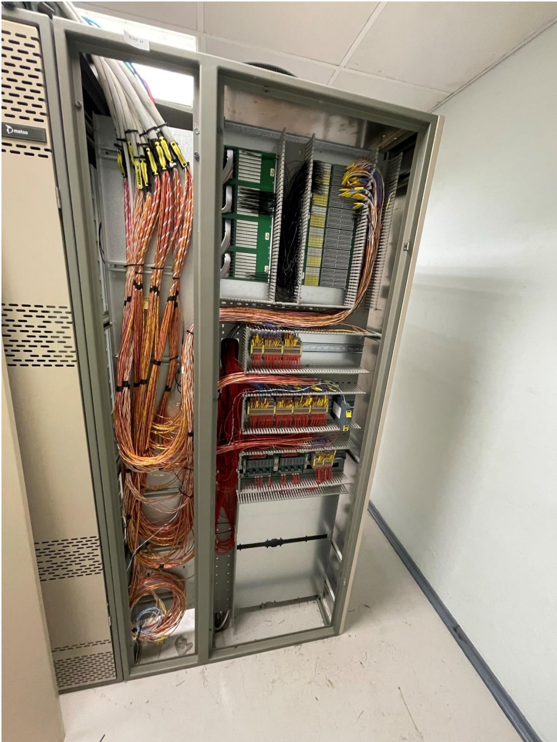
Figure 23 Water Heating Boiler 2 Cabinet Back
