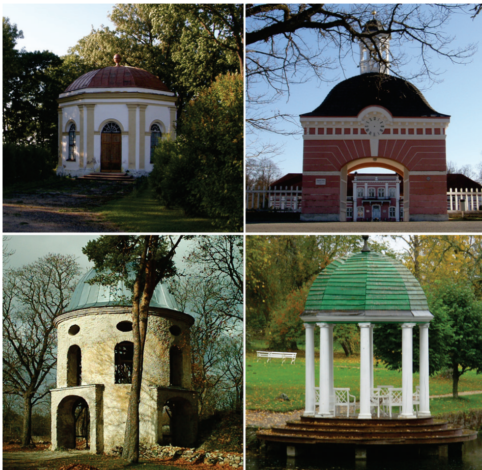
Figure 74. On the top left is a garden pavilion of Aa manor. On the top right is a gate-building of Sagadi manor. On the bottom left is a gate building of Sutlema Manor and on the bottom right is the reconstructed Palmse garden pavilion (photos by Sulev Nurme).
