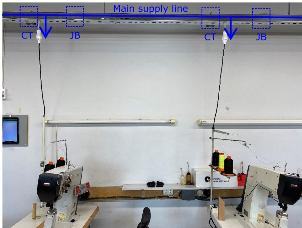
Figure 4.7. Current transformer installation at sewing machine (CT – current transformer, JB – junction box)
