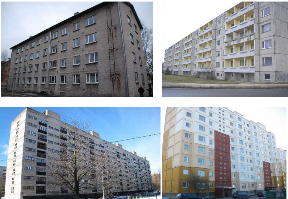
Figure 1. Example of studied brick apartment buildings (left) and panel apartment buildings (right).
