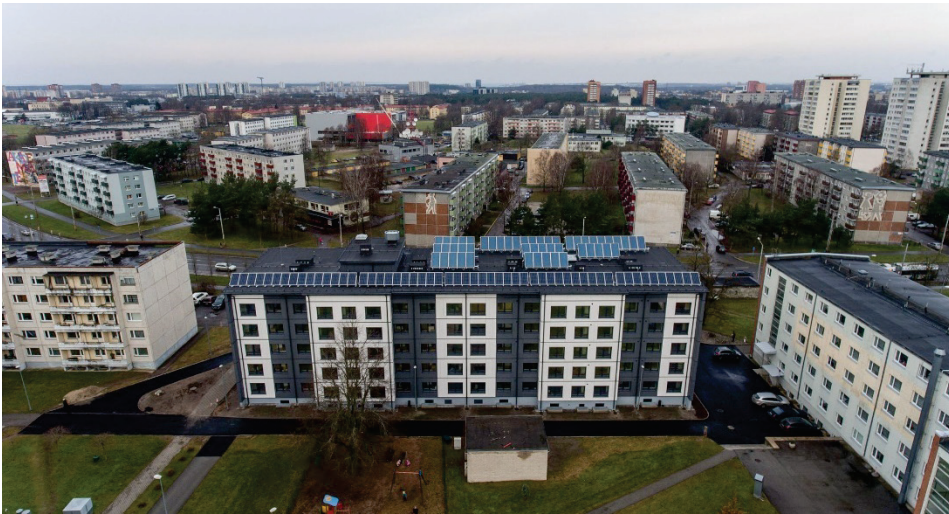
Figure 4.29 PCLP apartment building after renovation (Rudi 2017).
