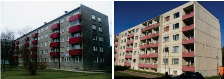
Figure 2.1 Examples of typical to Estonia PCLP apartment buildings, built in the 1960s–1970s (series 1-464, left) and 1980s–1990s (series 111-121, right). Photos from publications VI (left) and III (right).
