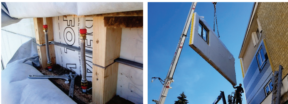
Figure 2.7 Integrated appliances in the elements (left). Installation of elements in the BERTIM project (right) (Lasarte et al. 2017).
