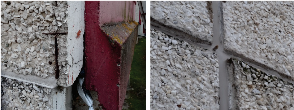
Figure 3.2 Facade details of the pilot building before renovation (2015).
