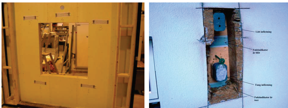
Figure 2.4 Testing of facade details in the project of insulation and technology procurement in laboratory (left) and on the plastered facade in Sweden (right) (Mjörnell 2011).
