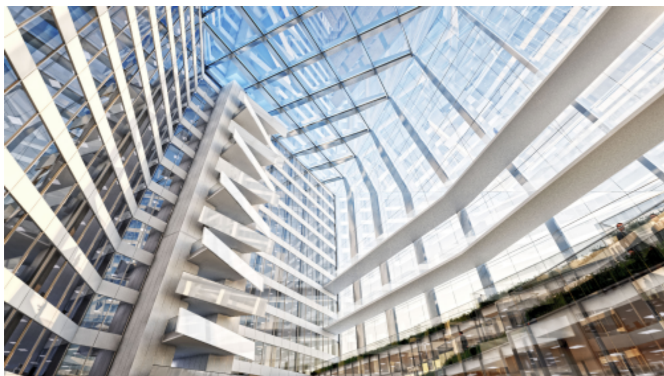
Joonis 10. The Edge - vaade aatriums https://thinkmarketingmagazine.com/edge-amsterdam-innovative-office-building-world/
