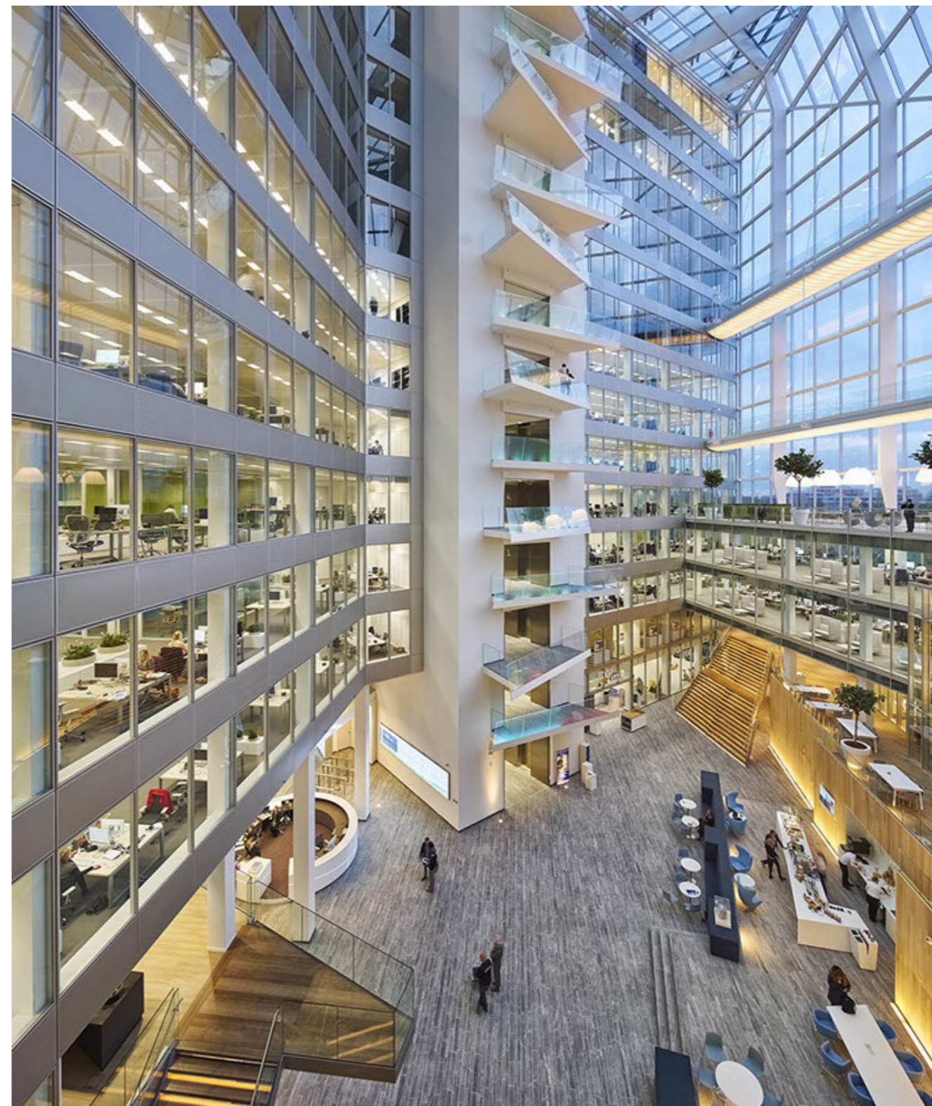
Joonis 11. The Edge - vaade aatriums http://www.plparchitecture.com/the-edge.html
