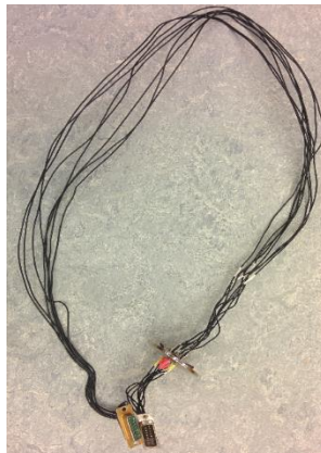
Figure 4-12 RMU power cable for vacuum test
