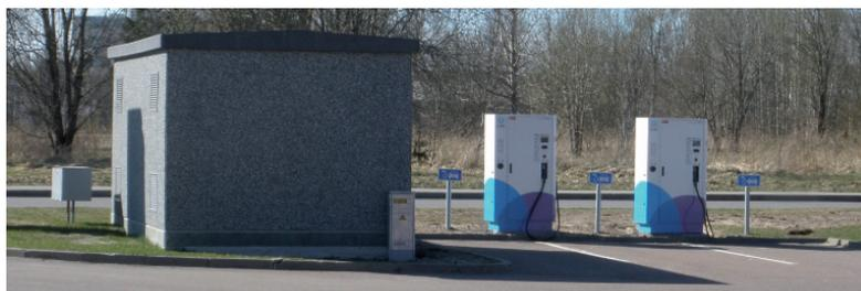
*Fig. 1.12 State of art – unidirectional ABB Terra 51 charge stations near a distribution substation*
