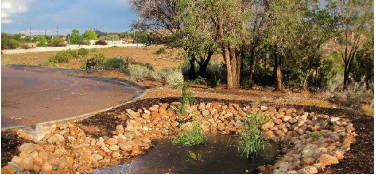
Pilt 7. Imbitiik. Ohio, Columbus (allikas: Southwest Urban Hydrology)
