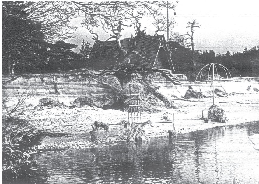
Photo 4. Extensive storm damage at the Järve-Keskranna lifeguard station in the February storm of 1990. (Photo – K.Orviku, 1990).
