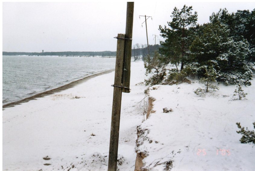
Photo 8. The January storm of 2005 damaged Järve–Mändjala sandy scarp to the extent of inclining the 32 kW poles of overhead line, providing the Sörve peninsula with electrical energy. (Photo – K.Orviku, 2005).
