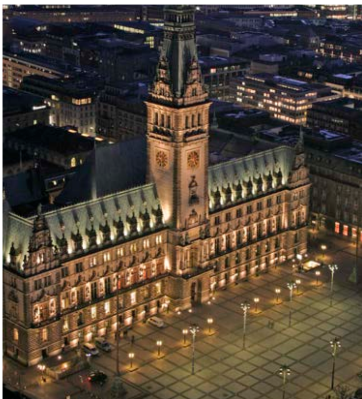
Figure 21. Illustration of a lighting strategy in action, wherein different zones are lightened as per different needs and purposes. Hamburg, Germany.
