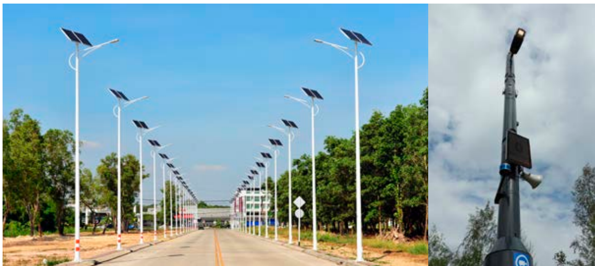
Figure 10. Real-life examples of smart lighting poles. Left: Energy-saving lamp post powered by solar cells. Right: example in the Baltic Sea region (Espoo, Finland): LuxTurrim5G Smart Pole 8 configured for traffic monitoring and public safety services: speed radar, 3D laser scanner, communication public address (PA) system and pole integrated information display.
