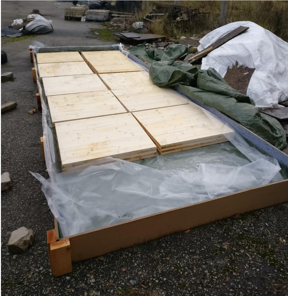
Figure 2.5: Arrangement of CLT panels inside the pool
