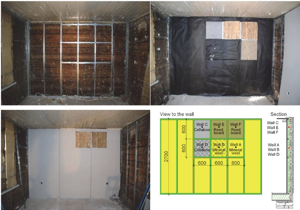
Figure 3.9 View of the wall during constructing the test walls construction and temperature and RH sensor positions on the log layer before the insulation material was added (bottom right).
