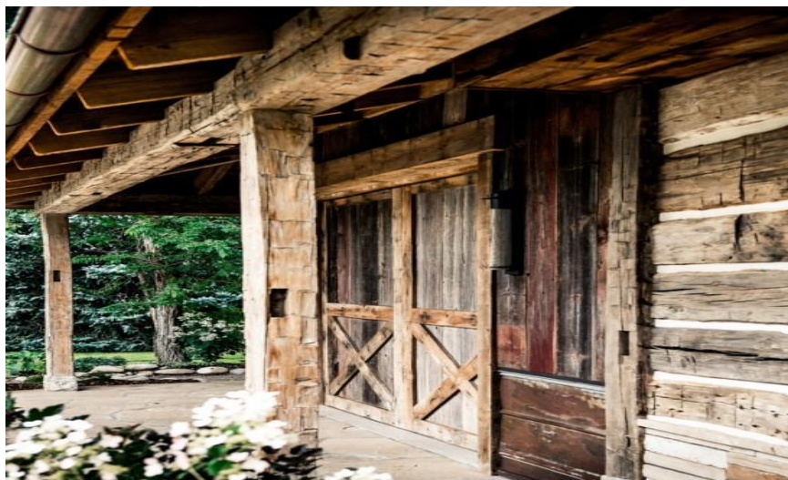
Figure 5. House of diverse hand-hewn types of wood. (Distinguished Boards & Beams, 2014)
