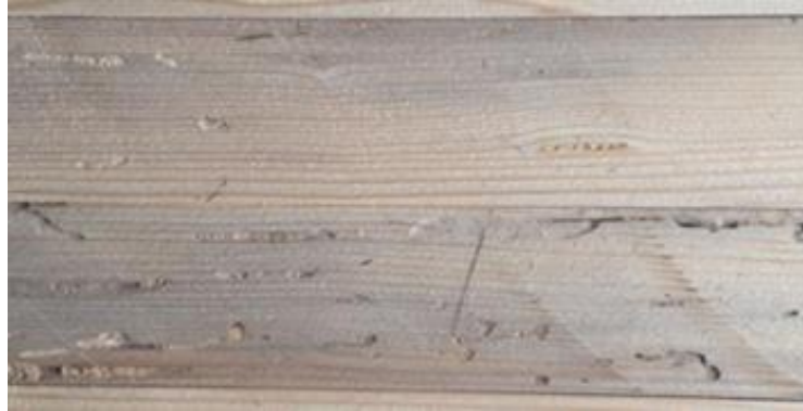
Figure 34. Boards inner conditions with insects damages.
