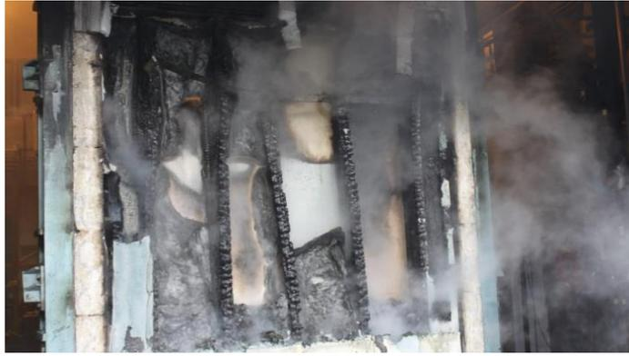
Figure 5.2-3 Buckling in walls plane after the fire exposure [9]
