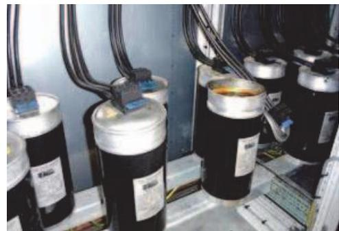
Fig. 2. Capacitor breakdown (on the right) due to high harmonic voltages in a LV system.
