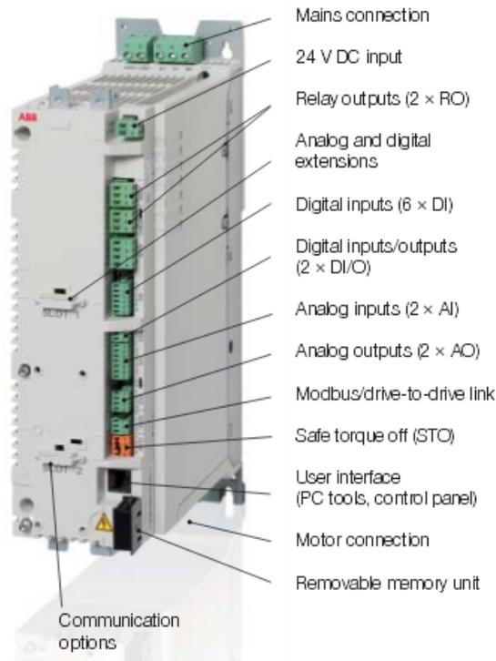
*Fig. 2.8 Interface connections of ACQ810.*
