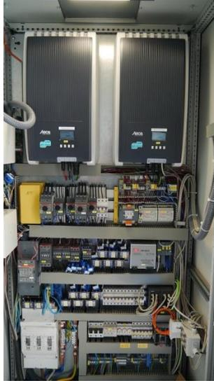
Figure 3-3. PV inverters and the switch cabinet of the nanogrid.
