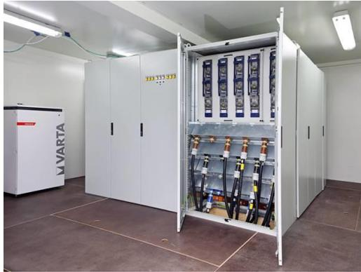
Figure 3-11. Switchgear.
