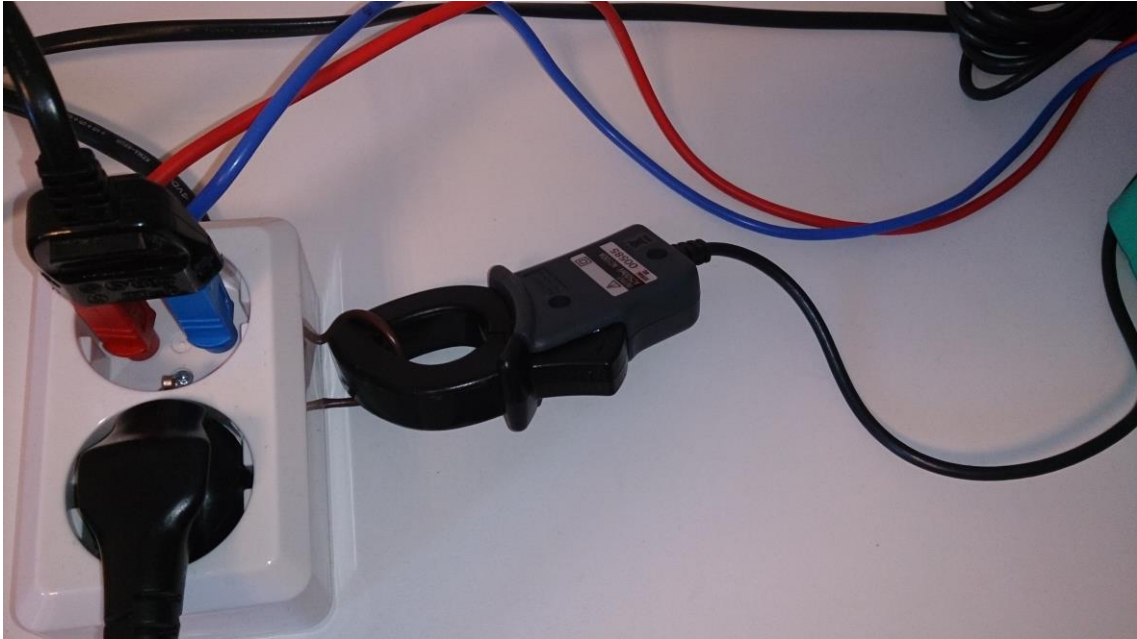
Figure 7. The voltage inputs plugged into the outlet and the current sensor.
