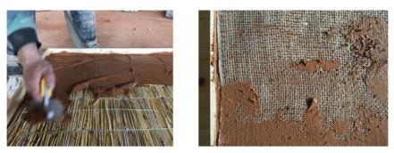
Figure 5-19. Plasterwork carried out in all test programs: Left – Application of a first plaster layer on a reed board; Right – Jute mesh applied on a plaster layer.
