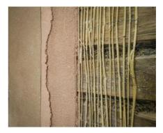
Figure 3-2. Examples of plaster support fixed on horizontal-log construction for the mechanical fixation of plaster: Left – Plaster applied on wooden lath and sticks. Right – Reed mat fixed to a log wall by using staples.
