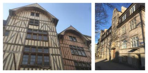
Figure 3-1. Different type of timber constructions in Europe: Left – half-timbered buildings in Germany; Right – Wooden apartment buildings in Estonia.
