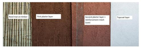
Figure 5-3. An example of a plaster system on timber element.
