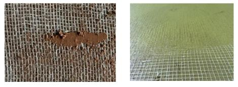
Figure 3-4. Application of reinforcement mesh into the clay plaster system: Left – Jute mesh; Right – Flax mesh embedded in the plaster.
