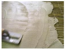
a) Application of the first layer of lime plaster using a trowel.
