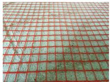
b) Glass fibre mesh on a lime plaster layer before the subsequent layer is added.
