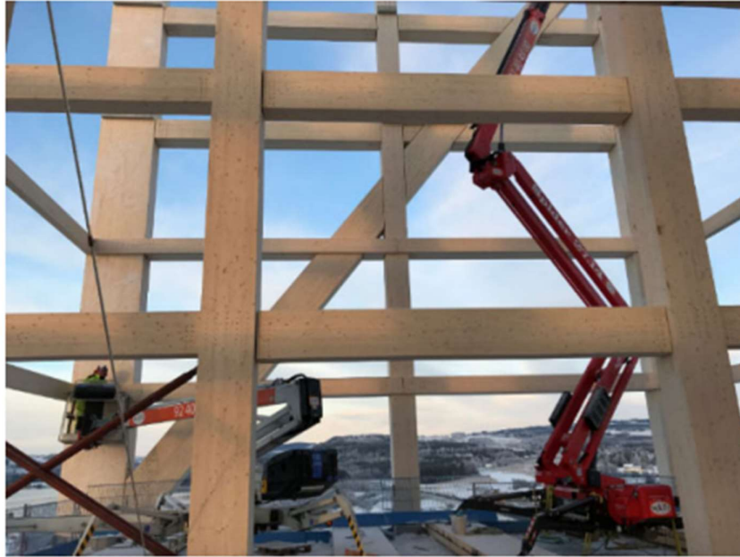
Figure 1.1 Glulam beams and columns
