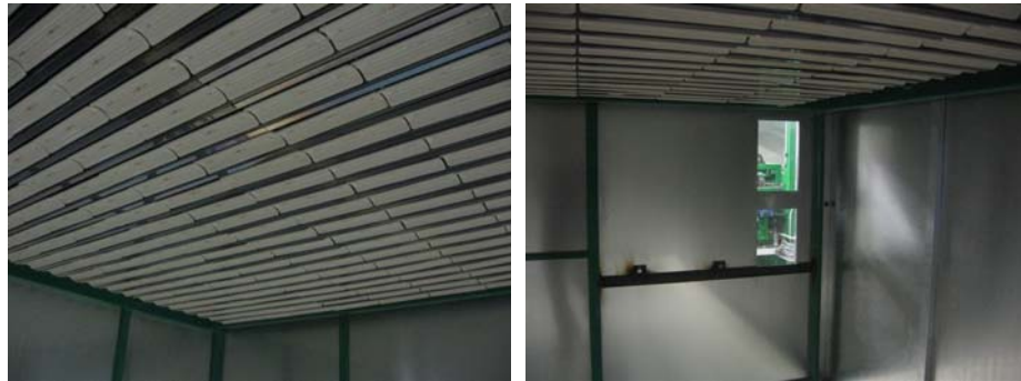
Figure 3.15. Infrared emitters in thermoforming bench
