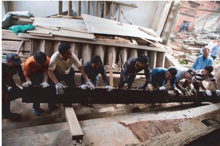
Figure 1. Volunteers working to move salvage crafted wooden pillars from the wreckage of Kasthamandap for proper storage (Source: Sandesh Munikar and Kasthamandap Reconstruction Committee).
